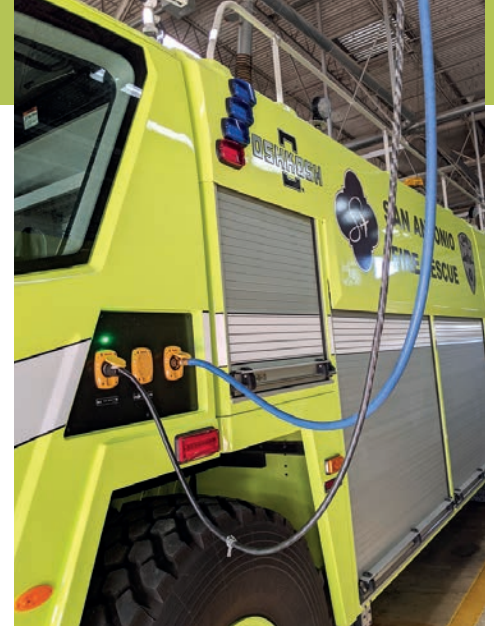
Truck stays ready hooked into shore power, connectors disconnect automatically when the truck moves out.
