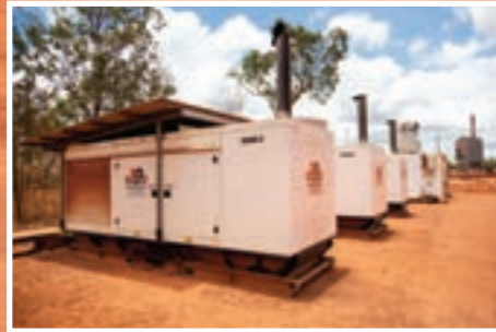
« The Scania R 730 pulls 210-tonnes without raising a sweat. Bauxite pebbles and ironstone chunks as found, far left. Canopies protect the Scania-powered electricity generators that keep the lights on and the AC running across the entire site.
